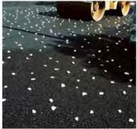
The Boulevard Garden, whose flooring is realized with a significant economy of means by mixing simple, almost trivial elements—like asphalt and white pebbles—to generate rich textures.
